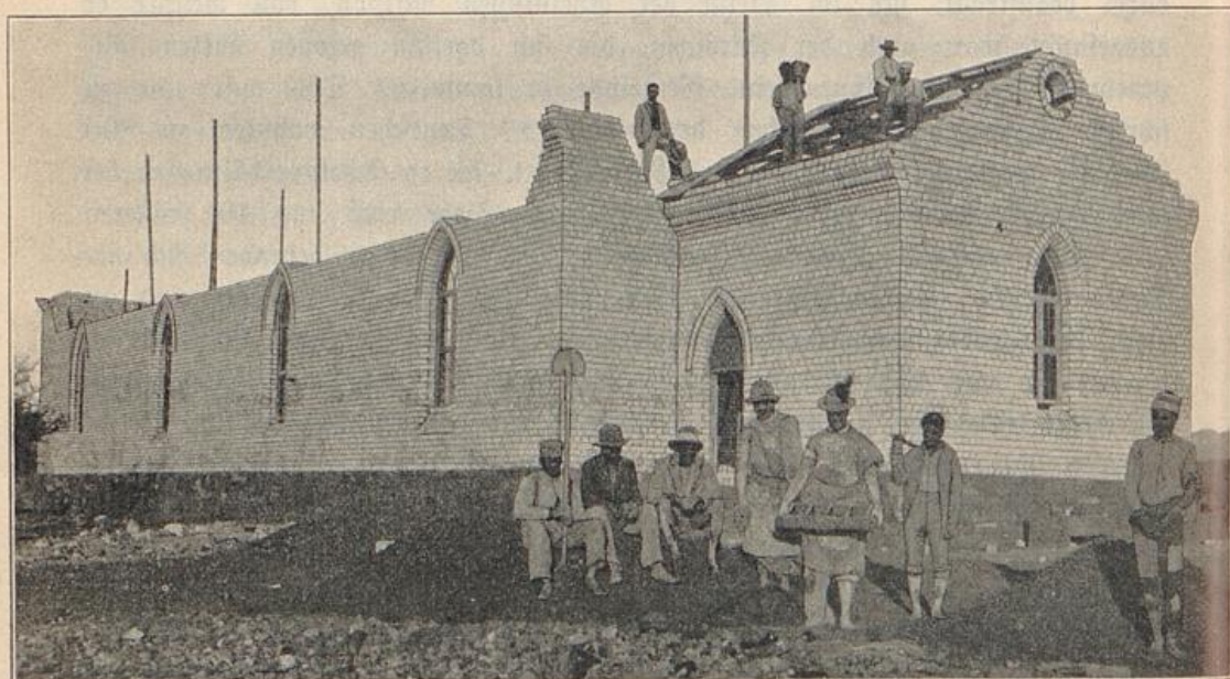
Kirchbau in Windhut.
