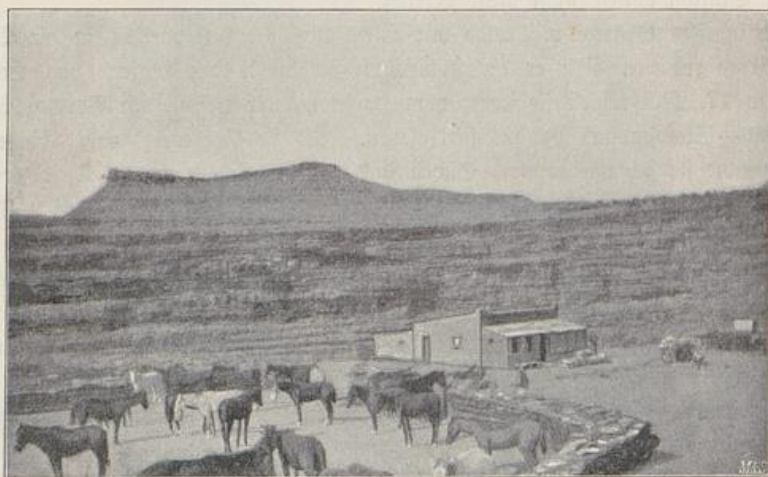
Station Haiams am Baiweg.
