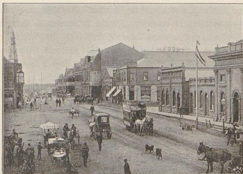
Rissick-Street in Johannesburg.
