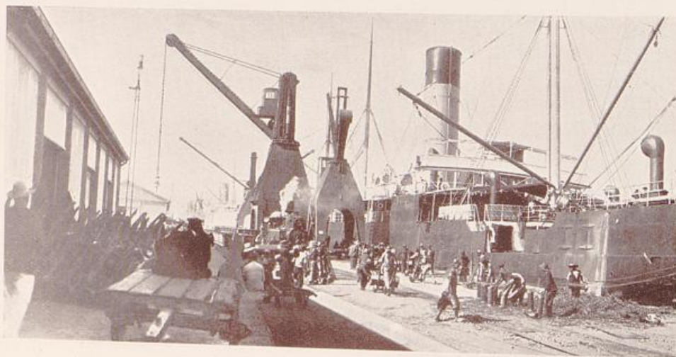
Paul's Wharf, Central (showing 50-ton hydraulic crane)
