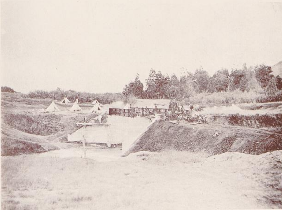
Ingoogo Bridge after lifting No. 5 girder, with Hart's River Bridge in the distance, Feb., 1910. Built by P.W.D.
