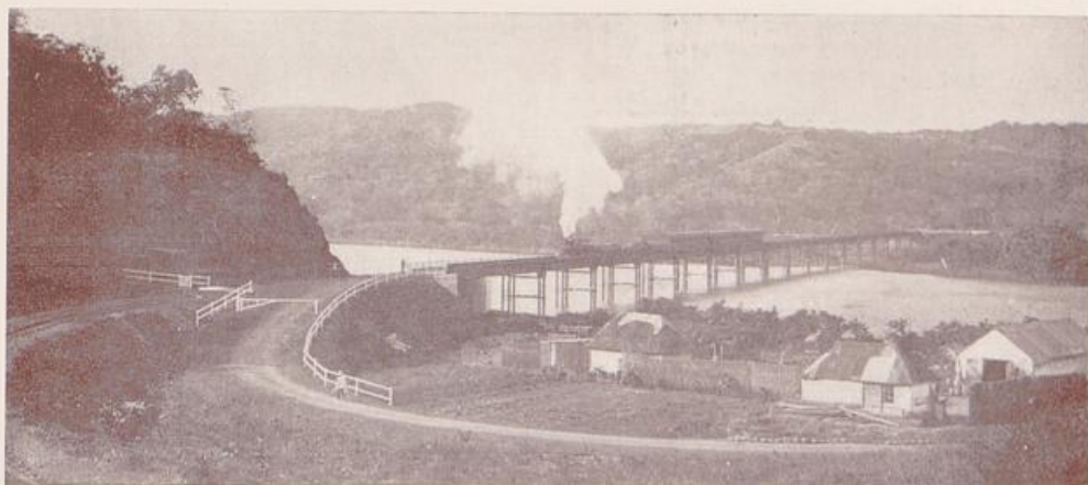
Umzimkulu River Bridge, Port Shepstone
