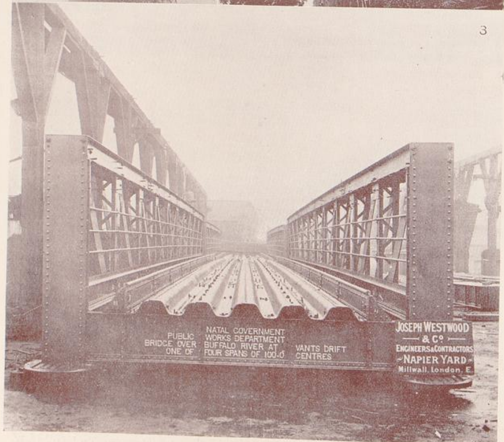
1.—Constructing Inuogo Bridge; No. 3 girder ready for lifting into position 2.—Reinforced Concrete Bridge, near Pinetown 3.—Span of Vants Drift Buffalo Bridge
