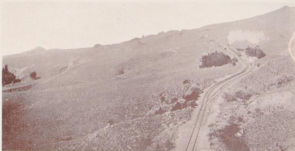
Reversing Stations, Harrismith Branch
