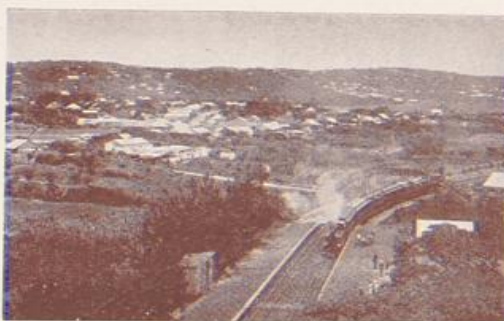
Berea Road Station
