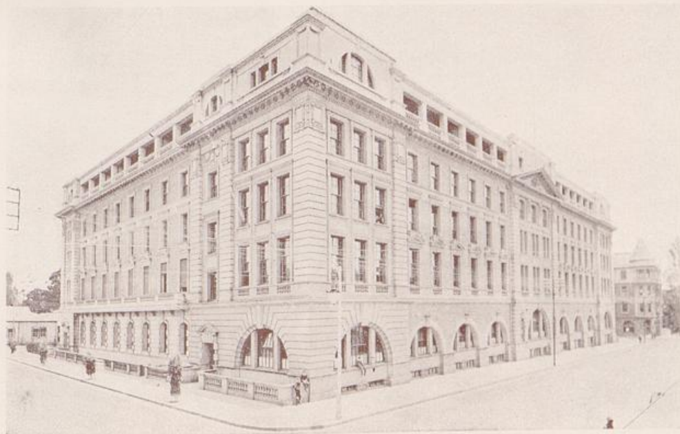
Headquarter Offices, South African Railways, Johannesburg
