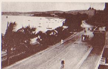
Bay Embankment, Durban
