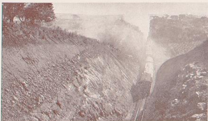
1.—Deep Cutting at Sea View 2.—Train passing through Fruit Farms near Bellair 3.—Road Bridge, Sea View
