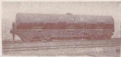
Cylindrical Water Tank.
