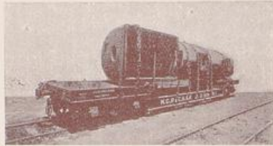
Well Wagon (Joint stock) loaded with boiler.
