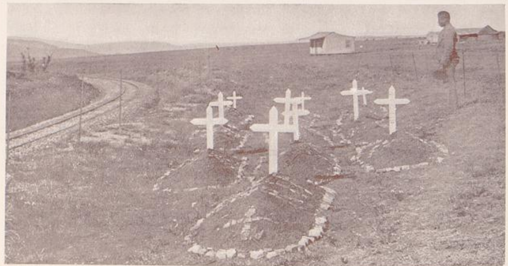
Graves alongside Railway Line at Glencoe Junction
