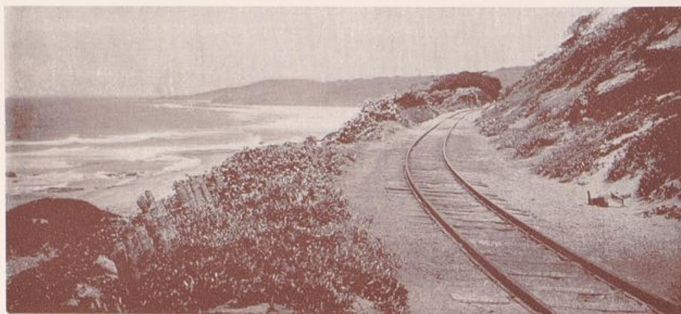
Railway Line at Widenham
